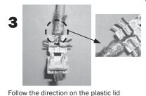
Follow the direction on the plastic lid color-coding to position T568A or T568B wiring, seperate a little space on proper position an dinsert the wire pair by pair into each slot.
