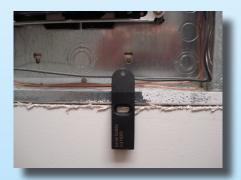
After removing the panel cover place the panel buddy on the edge of the panel in front of knockout to be removed.
