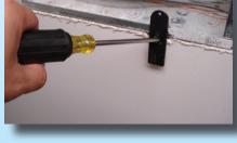
Next insert the modified screwdriver through the hole and between the drywall under the knockout.
