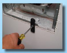
Push to loosen the knockout.
