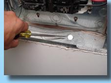
Using the screwdriver, remove panel knockout.
